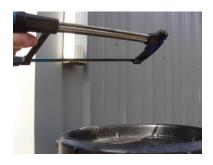
Cut your existing downspout about 6" to 12" above the top of the barrel
