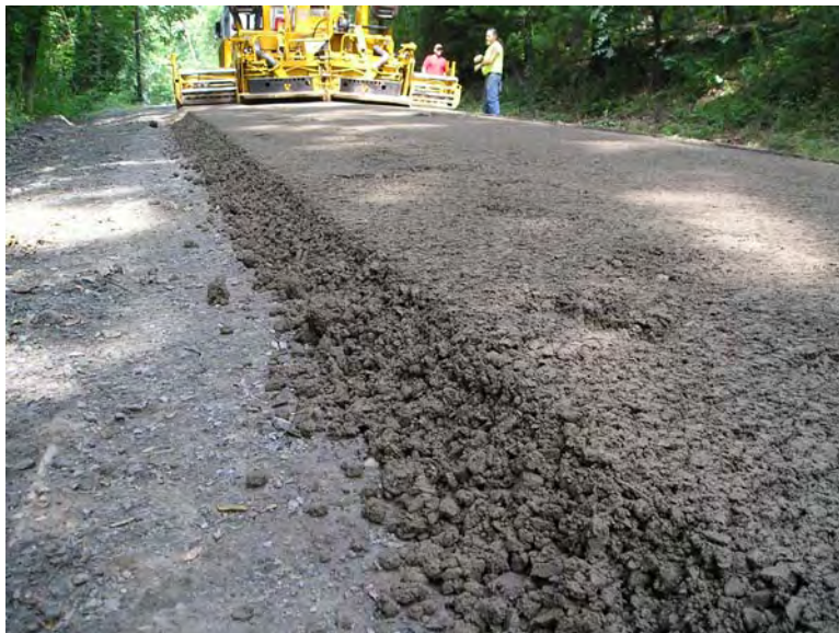
DSA is being applied using a paver.
