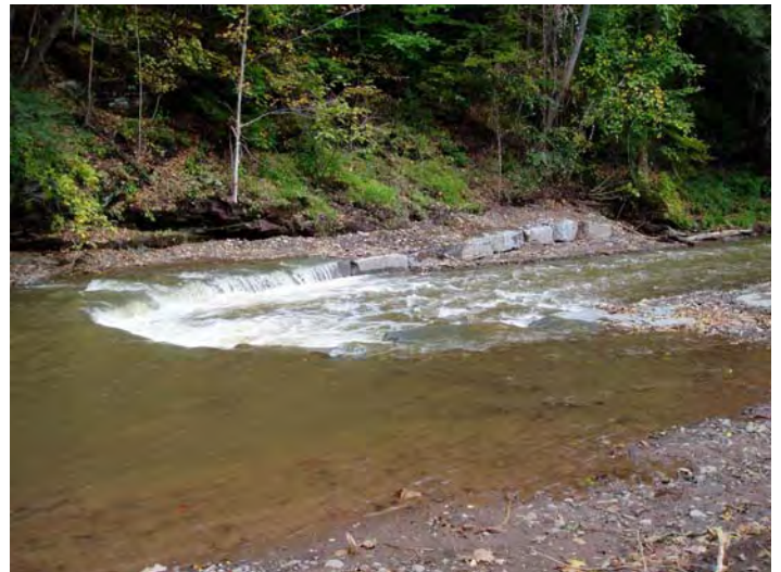
Rock cross-vane to control the stream's grade and flow.
