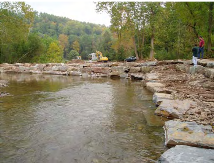
Channel plug to maintain stream channel dimensions.
