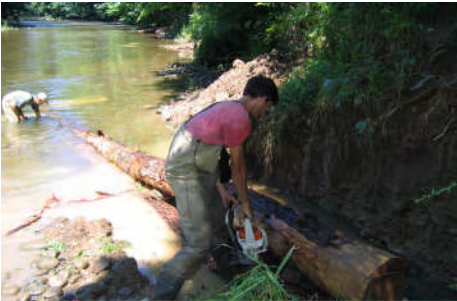
Multi-log Vane Construction
