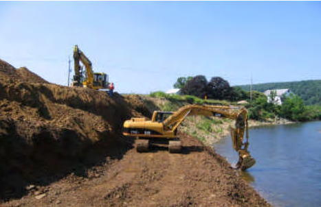
Construction of Bank Full Bench
