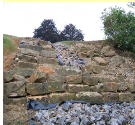
Constructed Head Wall at Downstream End of Project that Protects Previous Stabilization Work
