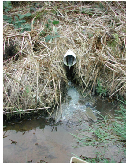
Failed septic system discharge
