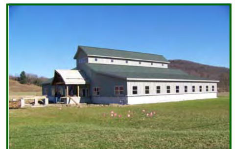
Education Center/Office Complex under construction
