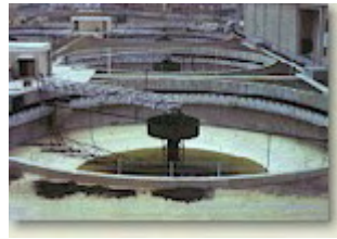
Wastewater Treatment Plant
