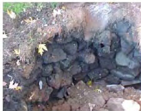
Figure 5. Collapsed Cesspool
