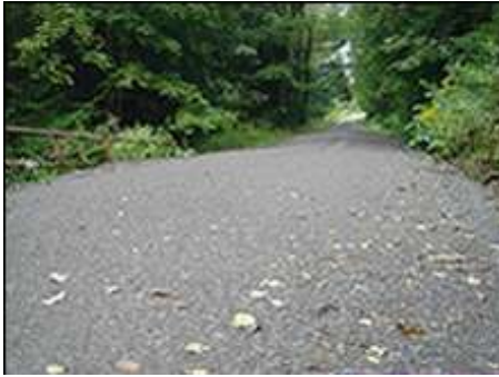
Driving Surface Aggregate is a mixture of crushed stone designed specifically as a surface-wearing course for unpaved roads.
