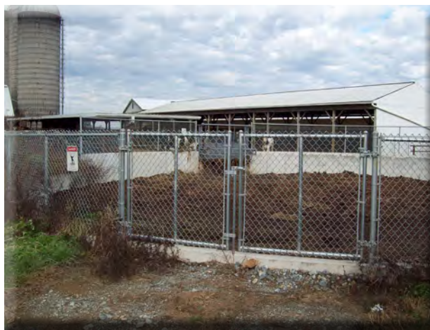
Properly installed safety features on a open manure pit.
